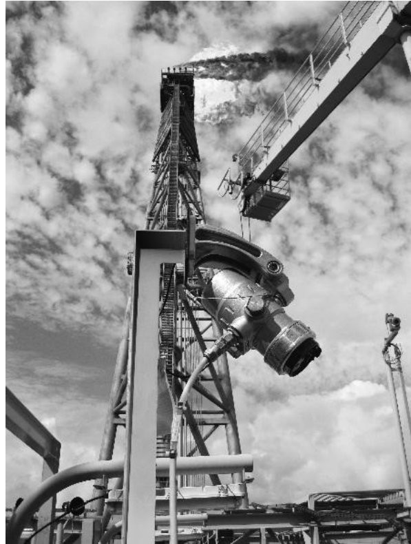
The detector pictured in center is a model X3301 multi-spectrum IR flame detector manufactured by Det-Tronics. This detector, mounted on an offshore oil platform, monitors the environment for IR emissions signals and outputs an alarm if the detected IR is consistent with an active flame. Pictured in the background is a flare stack used for burning excess or unusable product. The detector is pointed away from this flame source as it is not a fire of interest.
